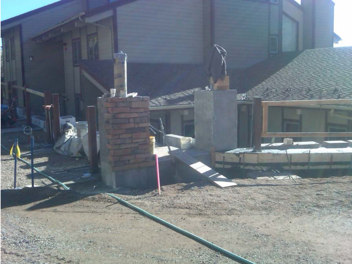
Stone at Stair Entry to Office
