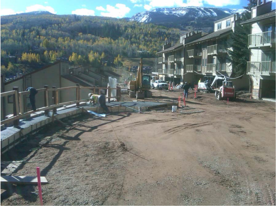
New Cement Sidewalk by Office—Road to Grade
