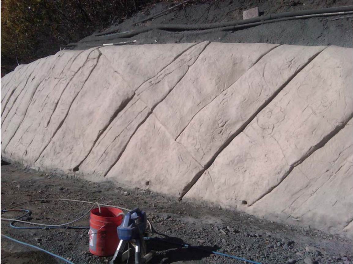
Wall by Entry to Complex
